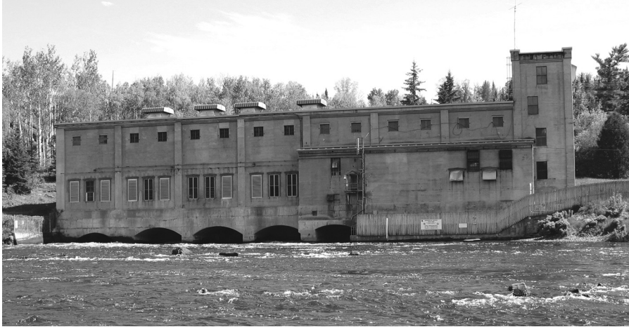
The powerhouse for the 24.6-MW Kakabeka Falls project was built in 1906 and expanded to its present size in 1914.
