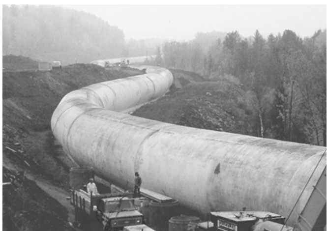
In 1998, a new single aqueduct capable of handling the maximum flow requirements for the station replaced the original three aqueducts.
