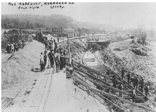
A third aqueduct was added to the 24.6-MW Kakabeka Falls project in 1914 to carry water to the new fourth turbine installed the same year.
