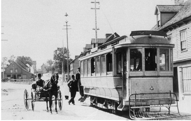
The Petty Harbour Hydroelectric Development began operation in 1900 to supply power to the St. John's electric street railway. When the railway began service, four streetcars served a population of about 31,000.
