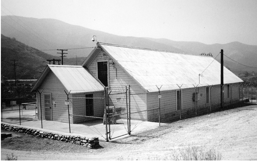
Because Southern California Edison's Mill Creek No. 1 hydroelectric plant is listed on the National Register of Historic Places, the powerhouse must maintain its original appearance.
