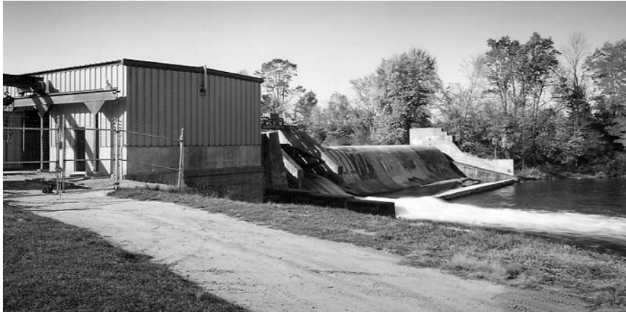
In the early 1980s, the exterior of the LaBarge powerhouse was modernized, and the original horizontal Francis unit was retrofitted. Today, the project—after 100 years—continues to generate clean, renewable electricity.
