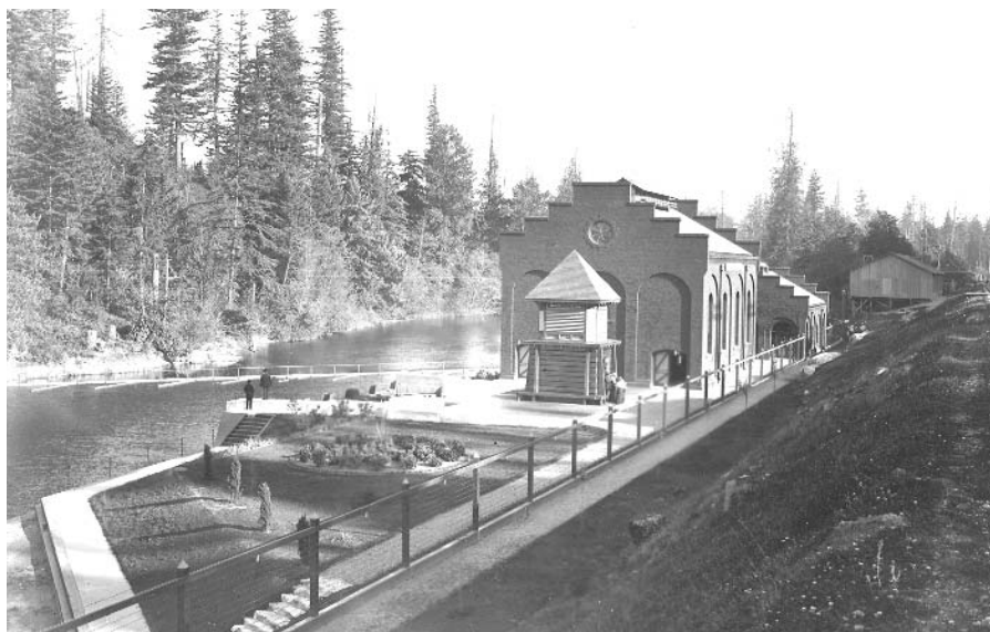
In 1900, the grounds of the Snoqualmie Falls Hydroelectric Project resembled a park, and the Transformer House was characterized by stepped end parapets, a gable roof, and tall, arched windows. The small building with the pointed roof housed the elevator to the underground generating station. (Courtesy Museum of History and Industry)
