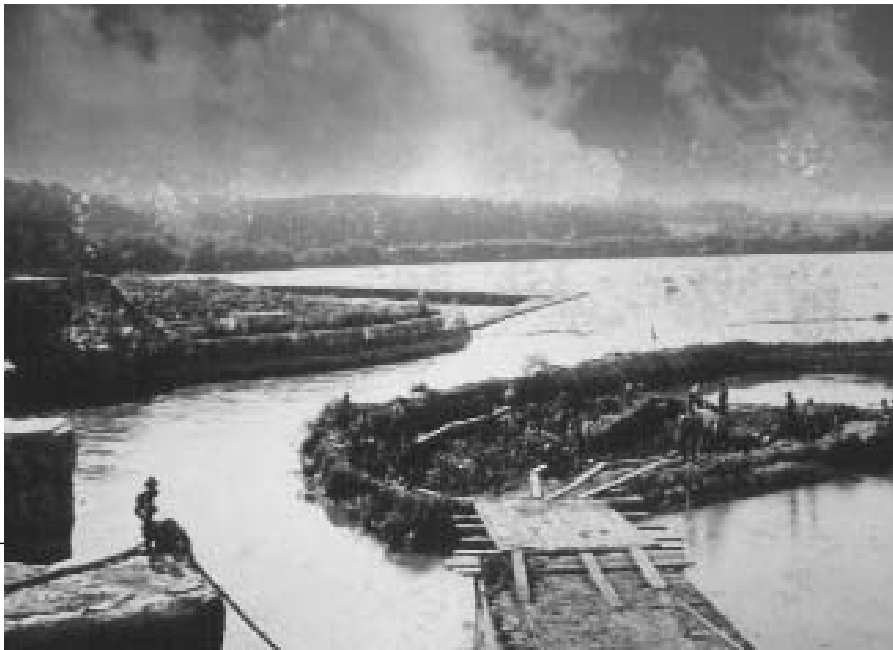
The state of South Carolina began construction on the Columbia Canal in 1819, in an effort to create a navigable waterway around the Congaree Rapids. The canal never did become a successful navigation route, but it did become home to the Columbia Canal Hydro Plant, which powered the first electric textile mill. A new powerhouse was built in 1896 and today still operates, contributing 10 MW to South Carolina Electric & Gas Company.
