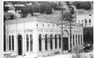
PacifiCorp's Granite Station turns 100 years old this year. This photo shows the 1.1-MW plant in 1915. (Photo courtesy PacifiCorp)
