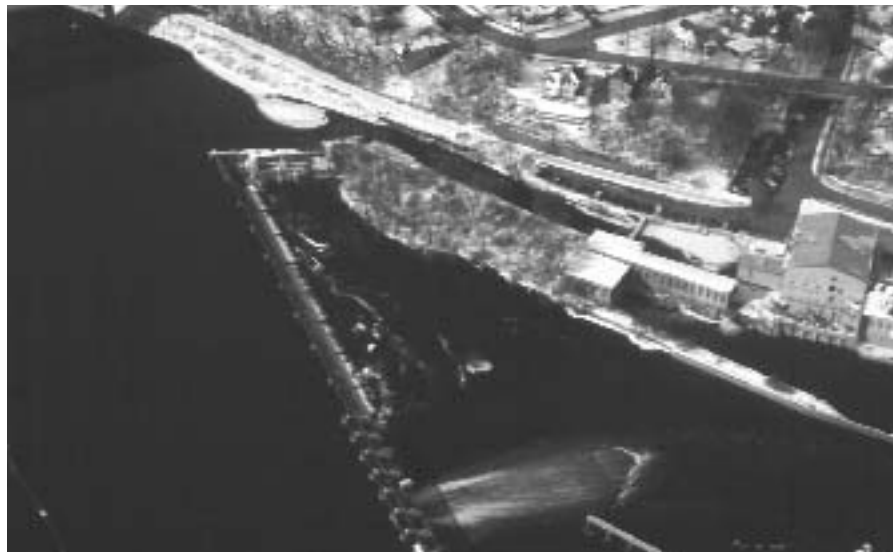
Site of Vulcan Street Hydroelectric Station, the very first hydropower plant. (Photo courtesy City of Appleton, Wisconsin, Department of Community Development)
