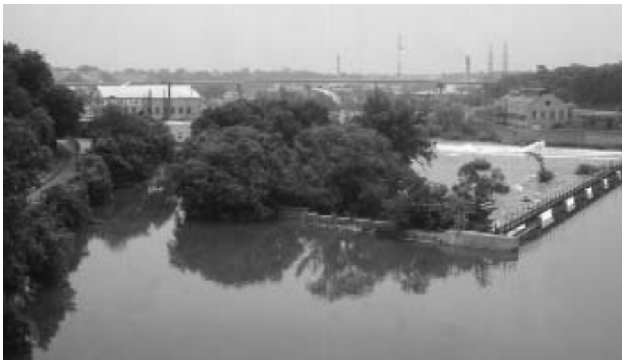
Kimberly-Clark operated the Vulcan project from 1908 through 1974. Among the properties that received power from the project was Kimberly-Clark's Atlas Mill, shown in the background of this photo.
